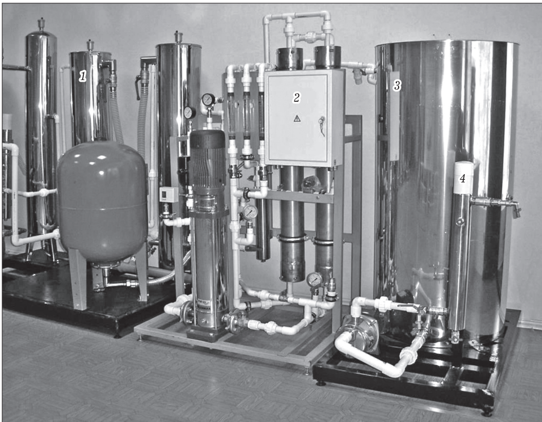
Fig. 2. Autonomous installation with the productivity of 0.5 m 3 /h for collective use: 1 – unit of preliminary water purification; 2 – reverse osmosis unit; 3 – tank for purified drinking water; 4 – ultraviolet lamp.
