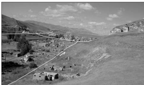
Fig. 6. General view of the Küçük Geçit village ruined by the 28 March 2004 Çayköyü (Aşkale–Erzurum) earthquake (view to west).
